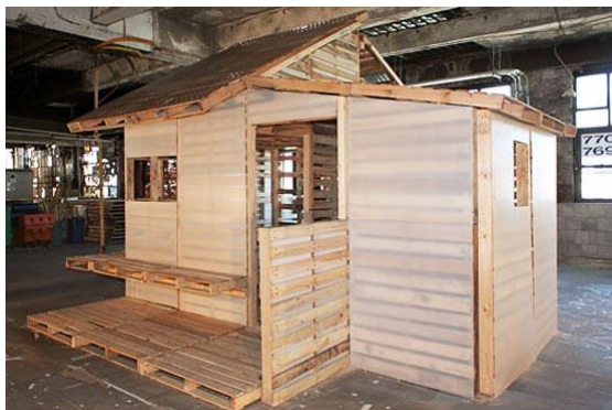
Figure 10. I-beam Palette House, housing for the returning refugees of Kosovo, Suzan Wines and Azin Valy
