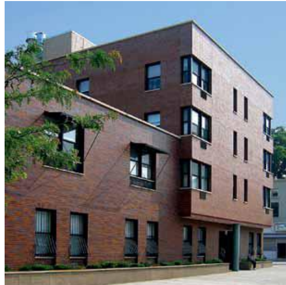
Figure 15. 614 Marcy Avenue, Brooklyn, 50 studios for formerly homeless, Jonathan Kirschenfeld Architects
