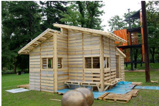
Figure 9. I-beam Palette House, housing for the returning refugees of Kosovo , Suzan Wines and Azin Valy
