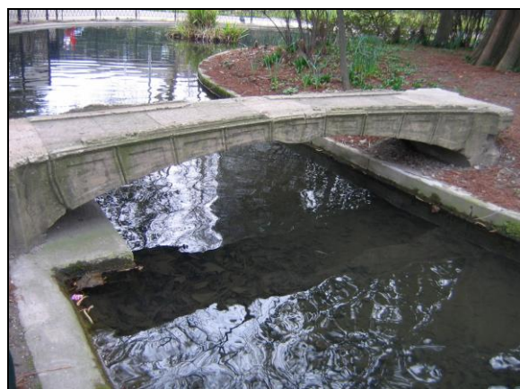
Fig.1. Reinforced concrete bridge, [8]
