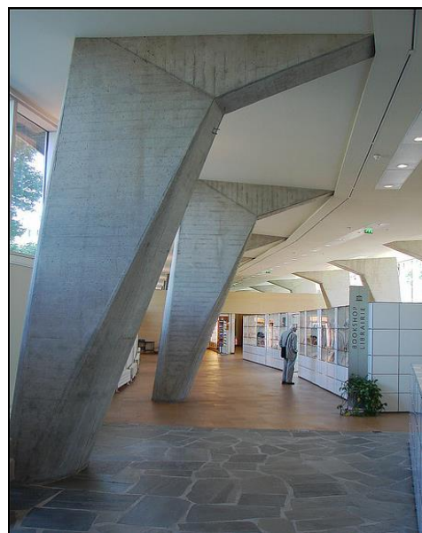
Fig.4 V shaped columns with cantilever, [6]
